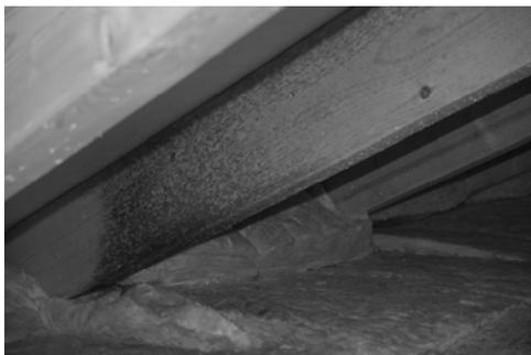
**Fig. 1:** Mould, caused by convective moisture transport from interior to cold roof
